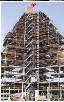
The largest scaffold ever - erected for a brown coal excavator - was a Scafom-rux SUPER 65/100 system, consisting of only a few vital but standard elements.
