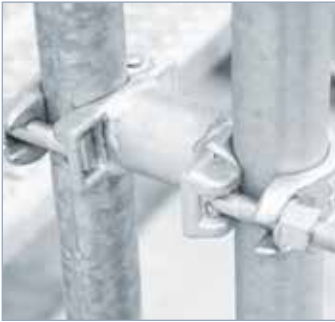
Bolted handrail holders
