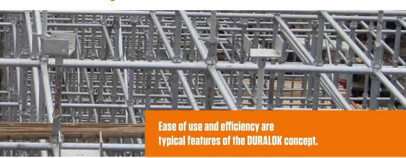
A single action fixes four components in one go. This means short assembly and dismantling times. A win/win situation!
